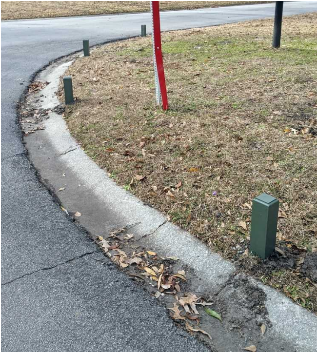
Typical Post Installation with spacing of 6' to 7' between posts
